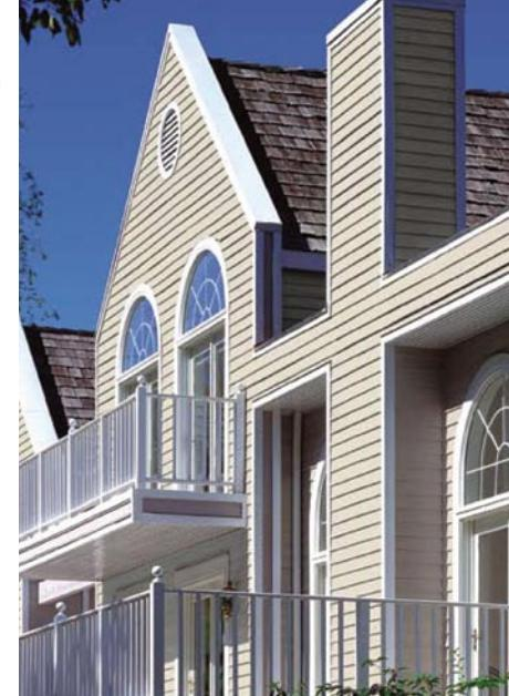
"A lot of guys out there working out of the back of their truck look for ways to cut corners," says Chris. "They just put new siding right over the old. We won't do that. First, we remove the old siding, then put up a Tyvek barrier. Finally we install a quality product from a quality manufacturer."
